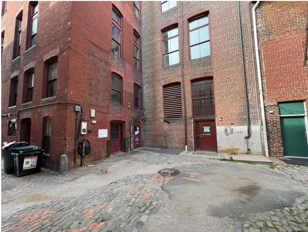
Photo-2 Rear of building 7 E Broad show exit doors from 5 and 7 side
