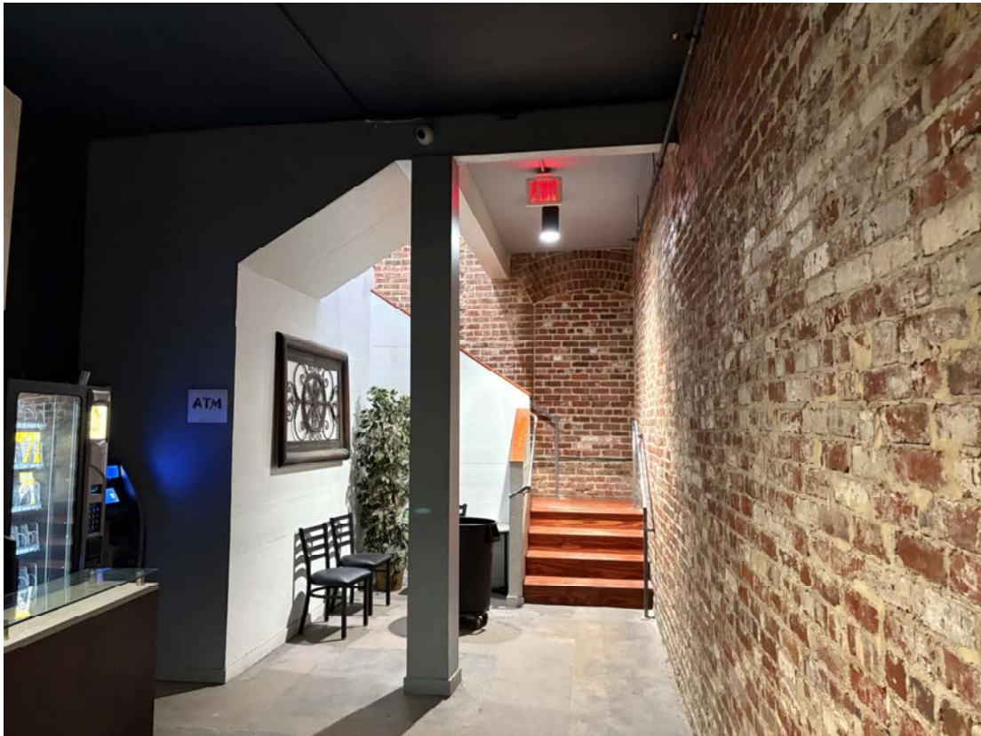
Photo-8 Interior Basement 5 side looking to rear exit stair
