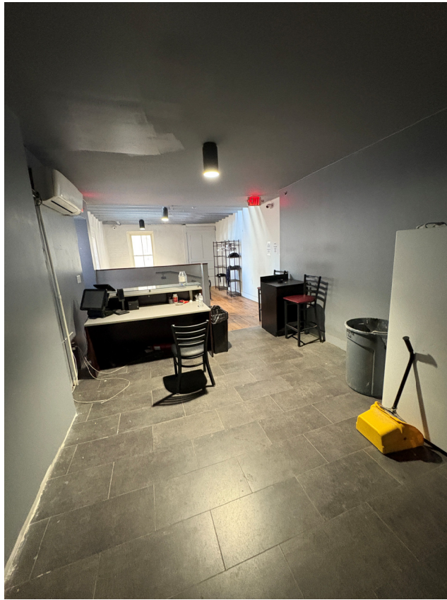
Photo-11 Interior 5 side Floor 1 rear exit to alley
