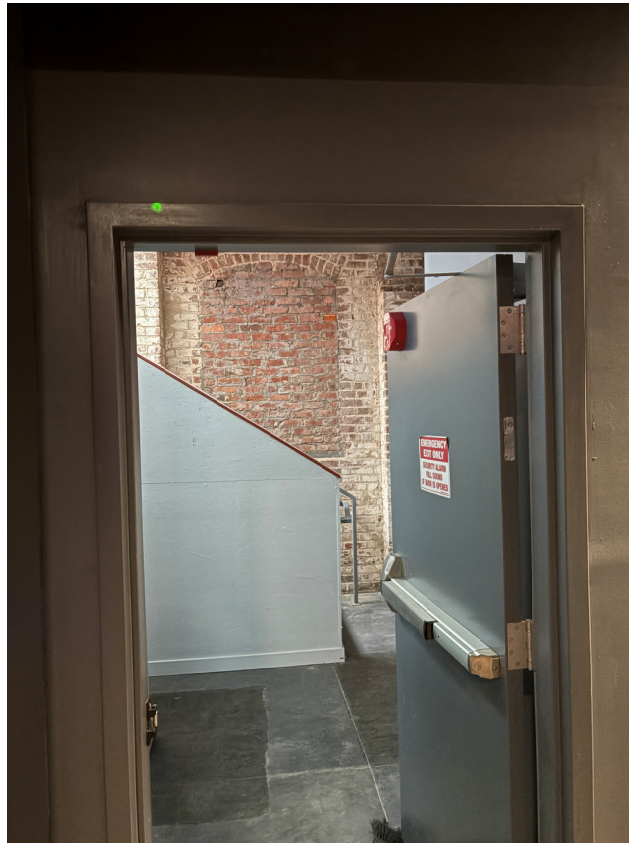
Photo-13 Interior Basement 5 side looking to front exit stair at Broad St
